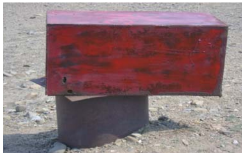
Fig. 16. Installed instrument for groundwater monitoring.
